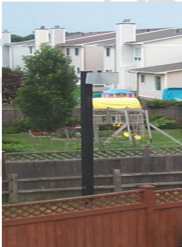
Shielding Solution for existing Street lamp – Kanata Ontario - 2003
