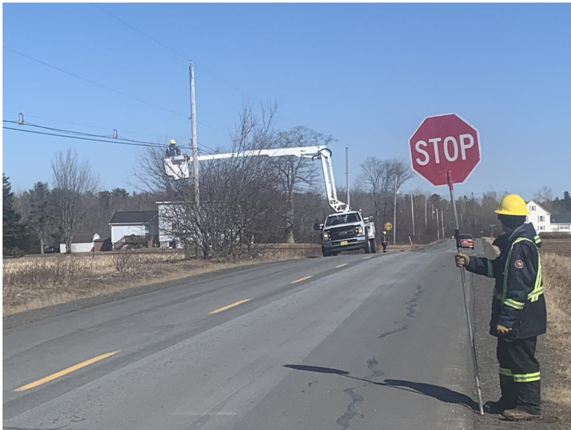
Fibre being installed in Kings County. More than 125 kilometres are now in place.
