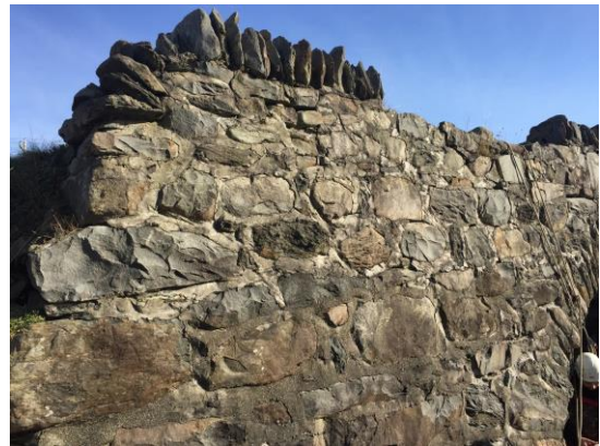
Figure 4: Partially tumbles south approach retaining wall (Left), Stones missing on west face of parapet railing (Right)
