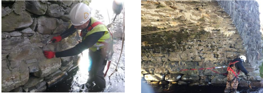
Figure 1: Testing of mortar deterioration (Left), Underwater video of arch foundations (Right)
