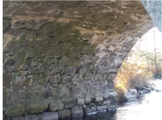
Figure 3: Deteriorating mortar on SE spandrel wall (Left), Presence of efflorescence on arch soffit (Right)
