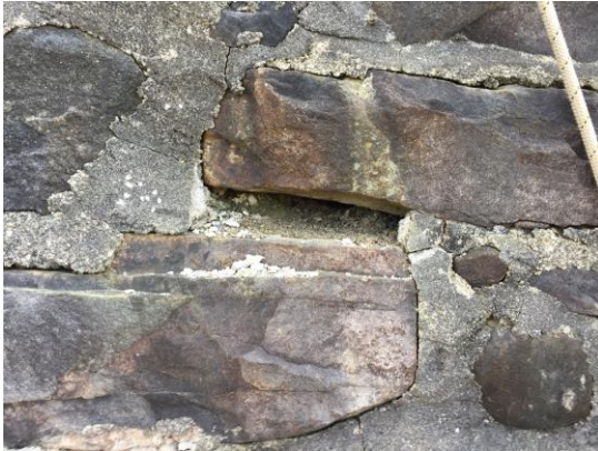
Figure 3: Deteriorating mortar on SE spandrel wall (Left), Presence of efflorescence on arch soffit (Right)
