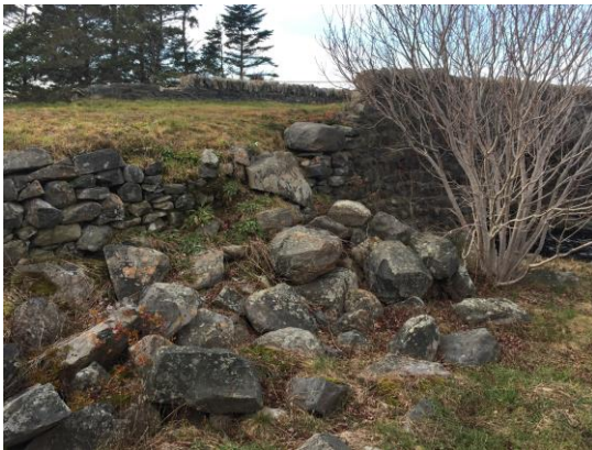
Figure 4: Partially tumbles south approach retaining wall (Left), Stones missing on west face of parapet railing (Right)
