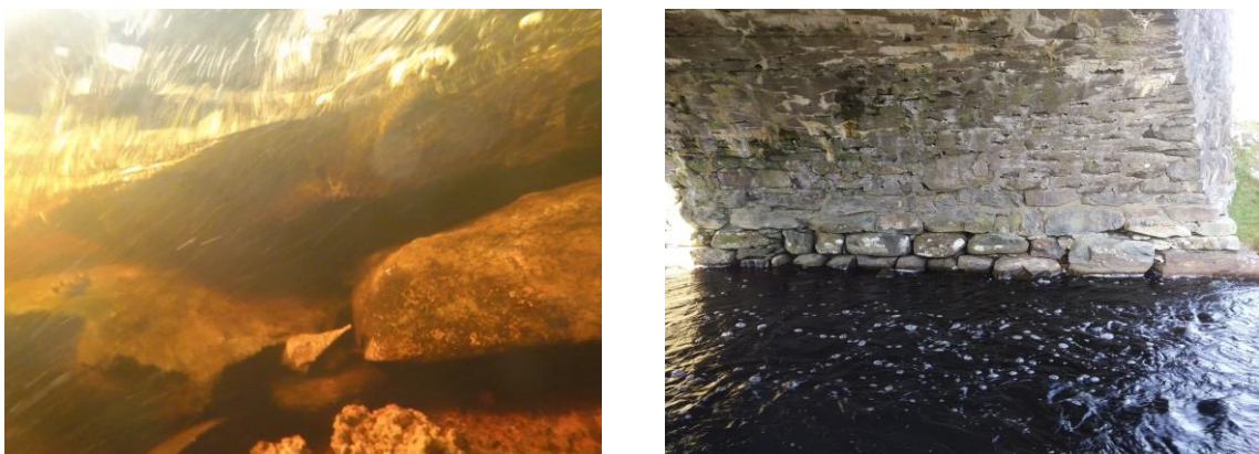
Figure 2: Loss of mortar in north foundation (Left), Condition of arch soffit (Right)
