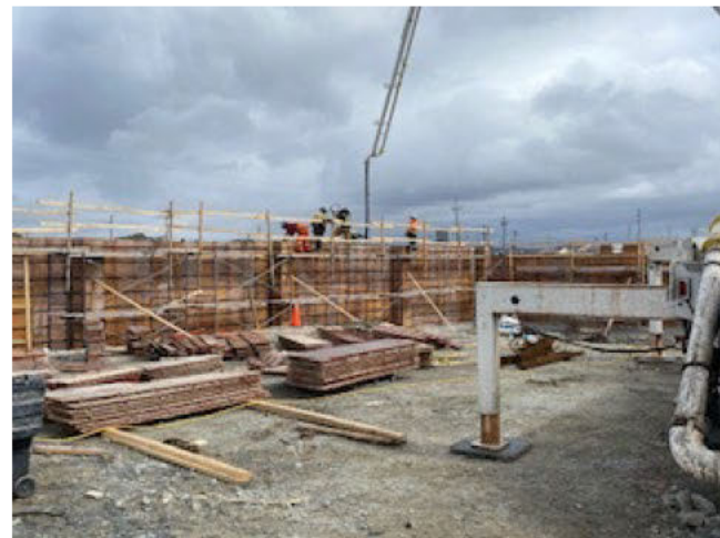
Figure 4: Concrete wall placement Grids L and 13
