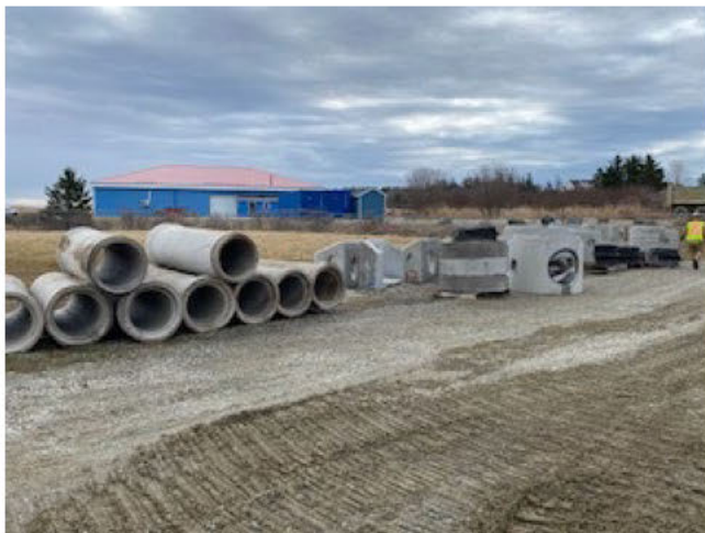
Figure 3: Manholes and storm pipe for site services
