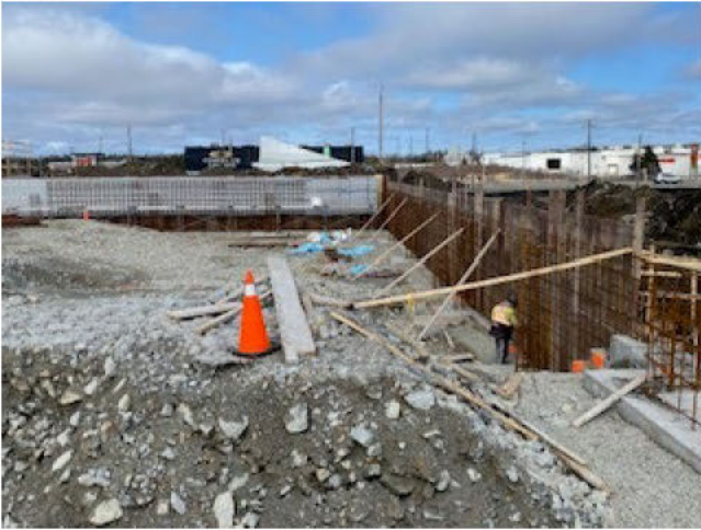
Figure 1: Formwork and rebar grid L and 13 foundation wall
