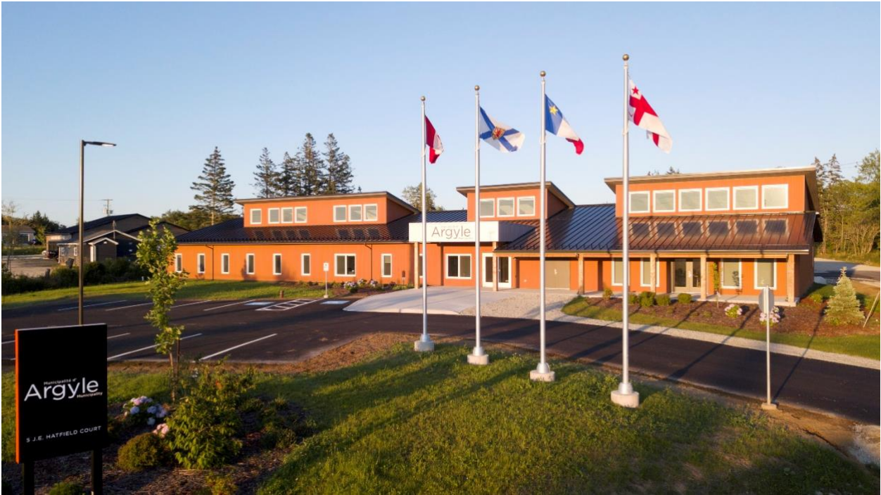
Figure 7: Municipality of Argyle - Net Zero Administration Building
